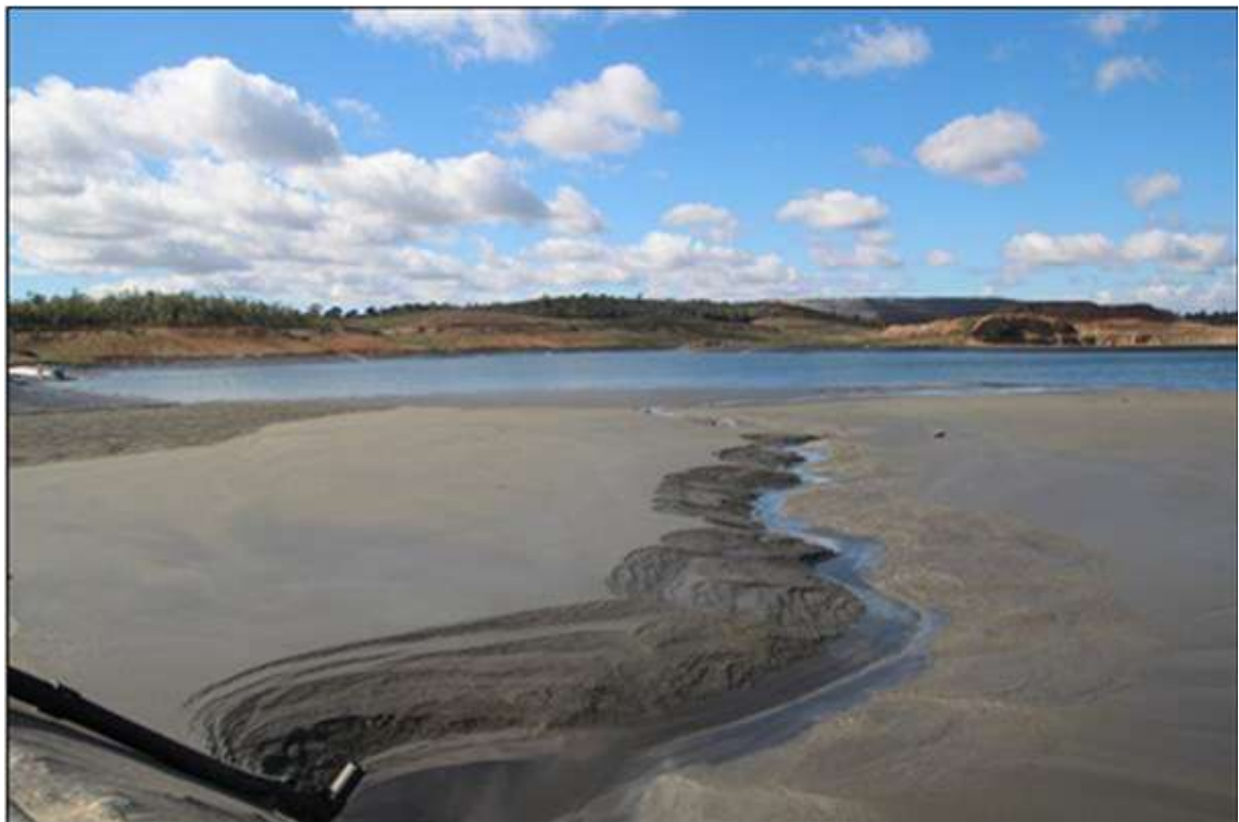
Figure 2.4: Beach made of extractive waste from mineral processing
