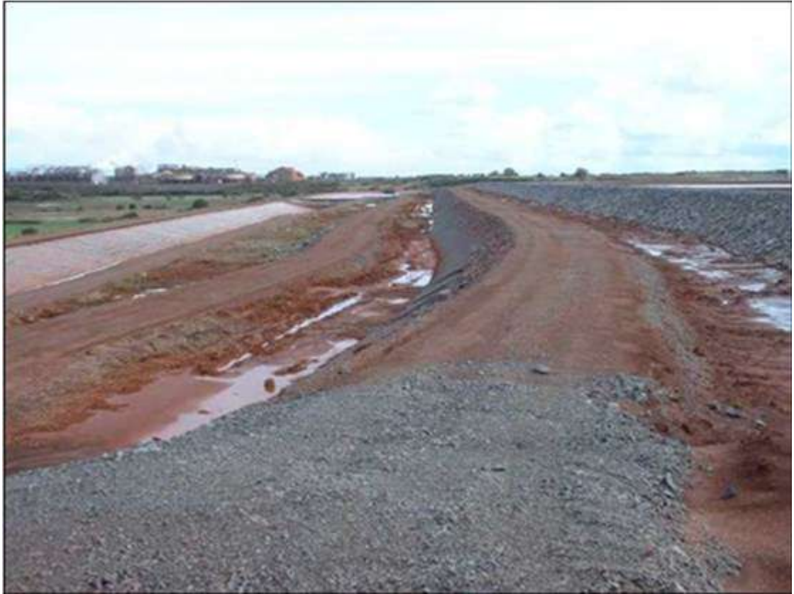
Figure 2.10: Dam raised using the upstream method at the Aughinish site
