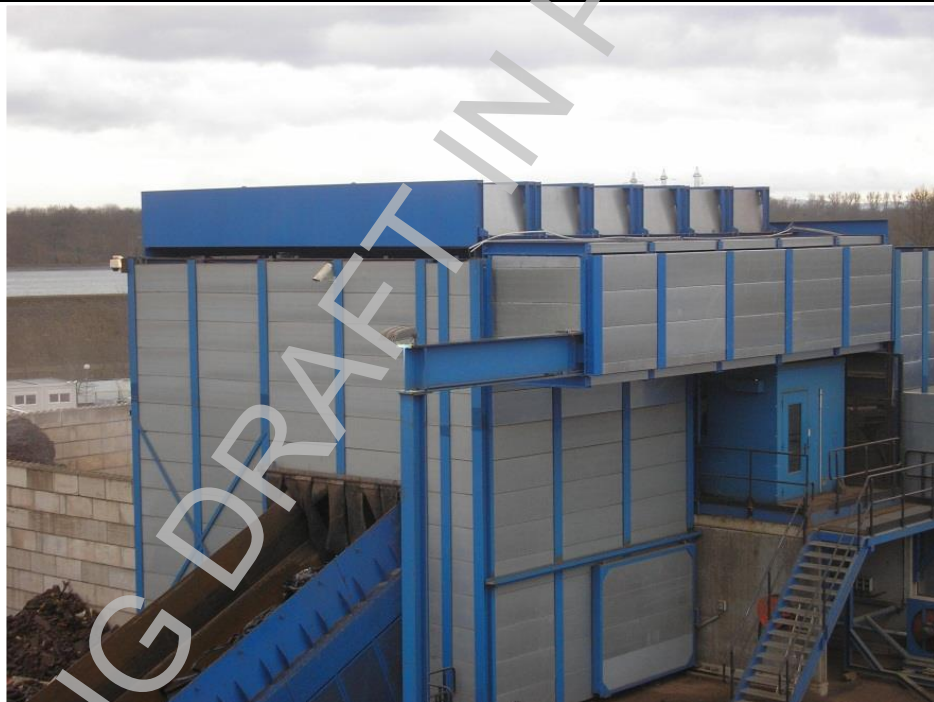
Figure 3.25: Splitter silencers at the roof of a shredding plant
