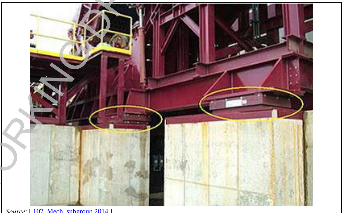
Figure 3.23: Isolation elements (circled) for vibration reduction
