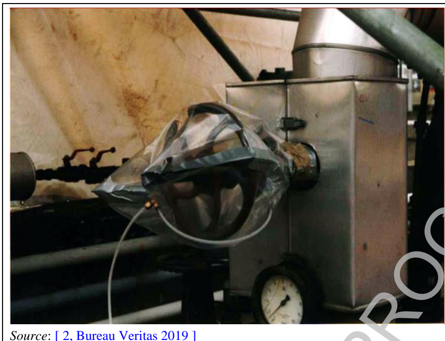
Figure 3.66: Bagging of a leaking valve
